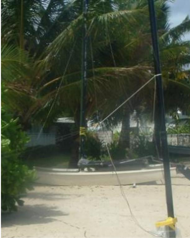
Once the 160/80 vertical was in place and the radials positioned oddly in/among trees with the two jackite poles (using only ~ 25') it was time for positioning the ends of the radials and doing a rough tuning. The 160 radials were trimmed and routed until a KAT500 tunable SWR was reached with the hairpin match. Then the 80 m radials were also trimmed and routed until the 80 m series capacitor, manually switched in, could get a tunable SWR on 80. Extra wire was carefully terminated at a tree.
