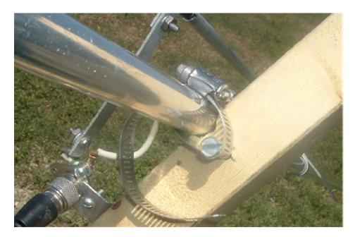
The gamma match is about 11" long with a 3 1/4" center-to-center spacing between the 3/8" gamma rod and the driven element. There is an bracket (insulated by electrical tape, probably not necessary and not touching the driven element) to hold the near end of the gamma rod in place.
